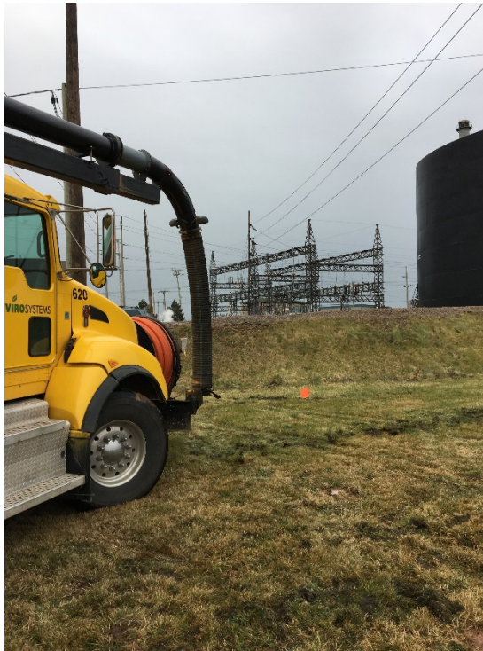
Photo 1 Hydroexcavating at MW-2, looking south.
