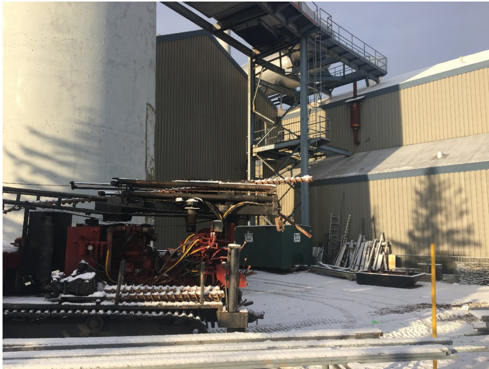
Photo 3 CME 55 track mounted drill rig setting up on MW-12, looking west.
