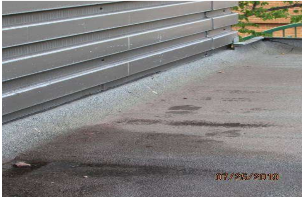
View of wall base flashing.
