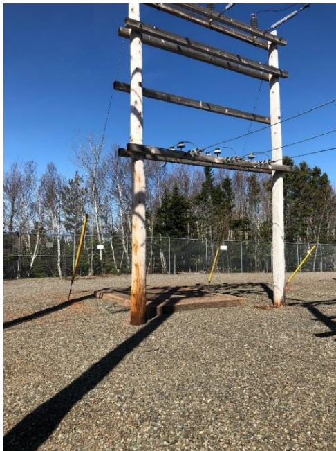
The bus structure (left) is measured to be approximately 12 feet above ground level (right). The new bus structure will be 25 feet above ground level.
