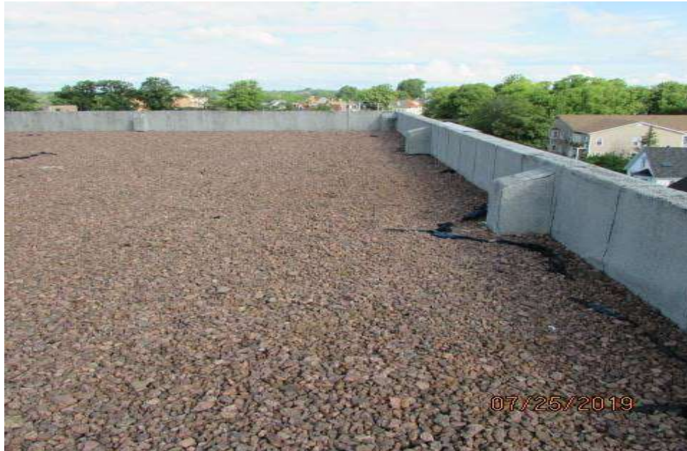
View of roof.
