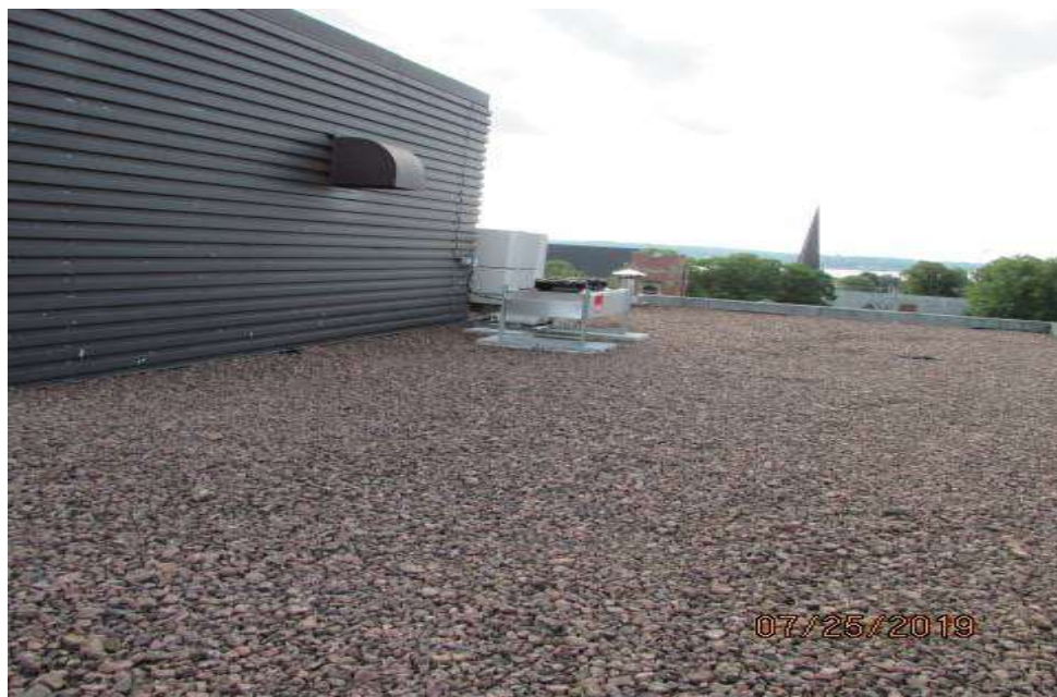
View of roof.
