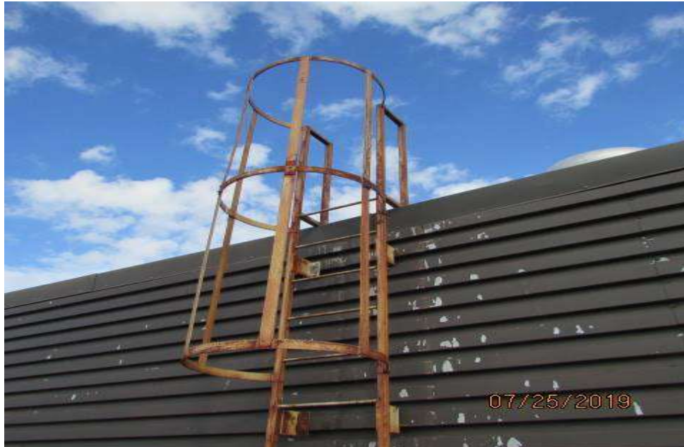
View of ladder to upper roof.
