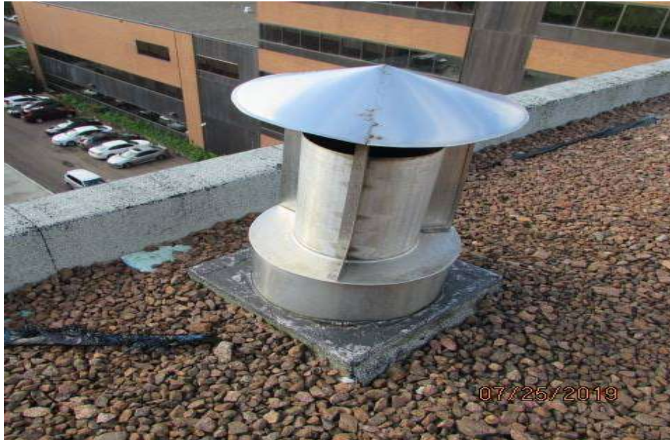
View of vent stack on roof surface.
