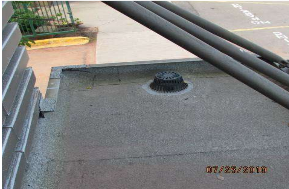
View of drain on south side of building.
