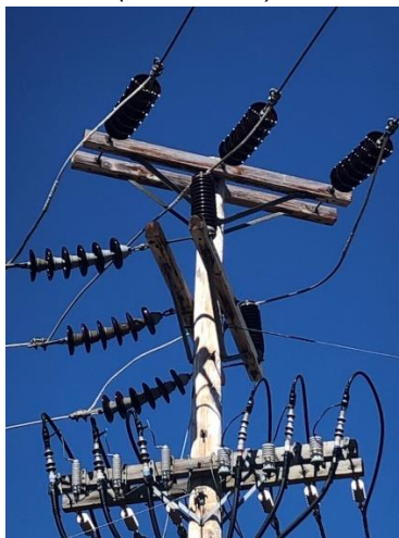
Aged and deteriorated crossarm structures.
