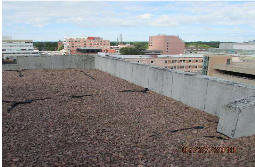
Exposed base flashing membrane.
