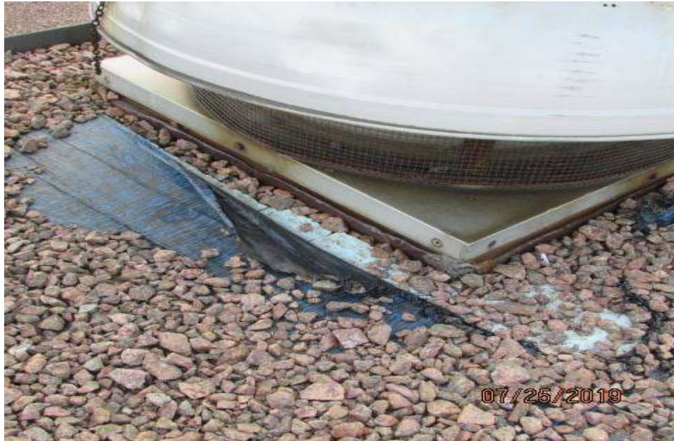
Ballast can get between the insulation and membrane. This can damage the roof membrane.
