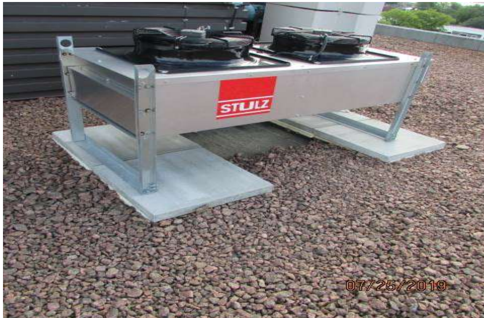
New roof top unit on roof surface.
