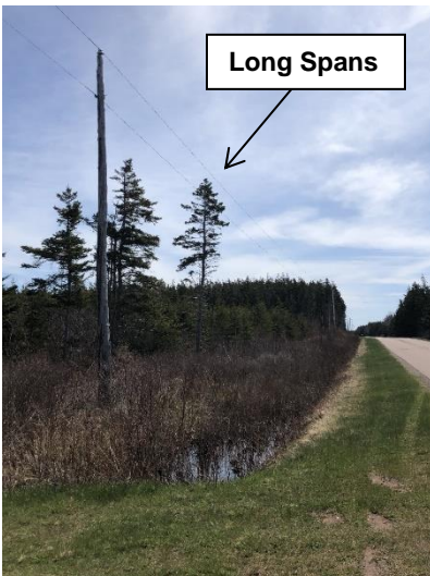
Eastern cedar pole with long spans
