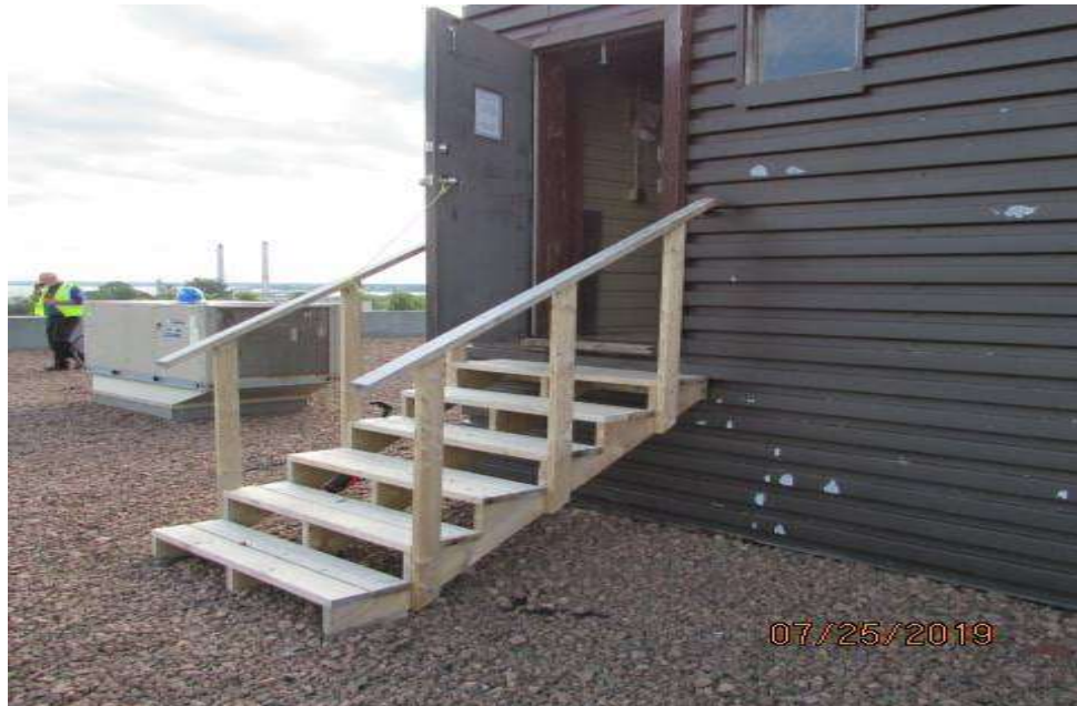
Stairs from roof entrance.
