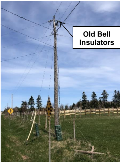
Eastern cedar pole with old bell insulators
