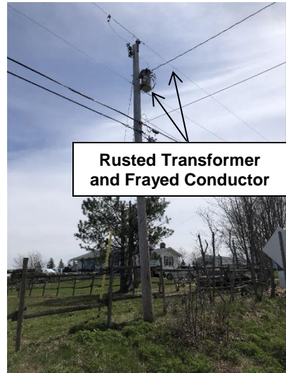
Rusted transformers and frayed conductor
