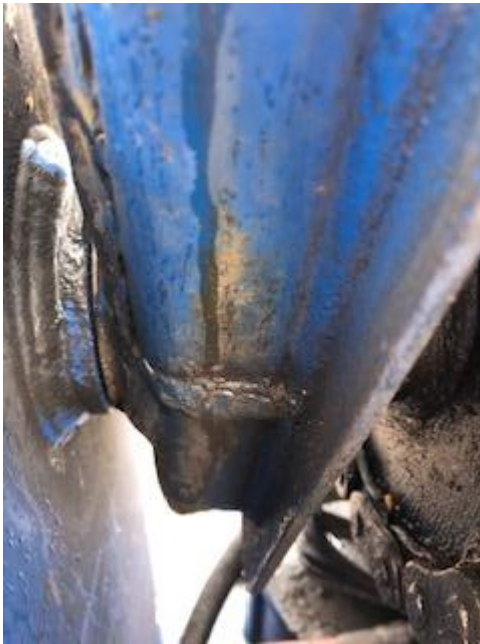
Truck 12-12-58 Weld repairs at main turret
